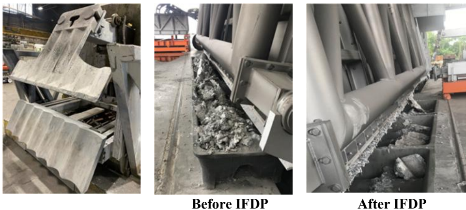
Figure 9. In-furnace dross processing skim and cold plate.
